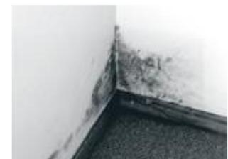
Condensation has led to mould Growth in a corner.
